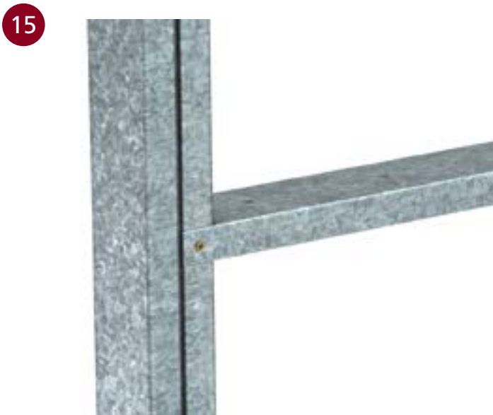
■ NOGGING TRACK FIXING DETAIL AT MAXIJAMB
