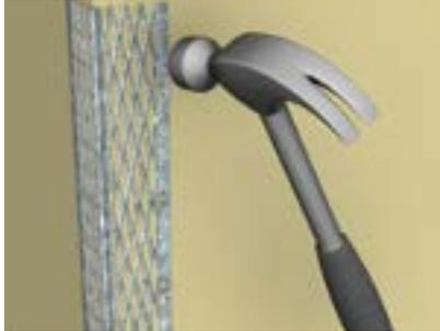
Beads can be attached by nails or a staple gun at not more than 500mm centres down the legs of the bead, and not more than 100mm from each end.
