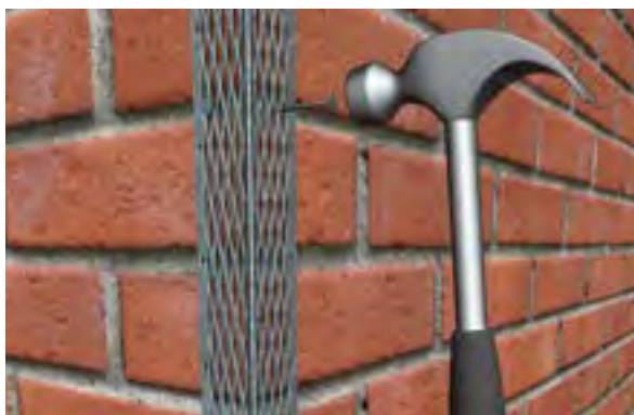
■ NAILING INTO THE MORTAR ON MASONRY WALLS
