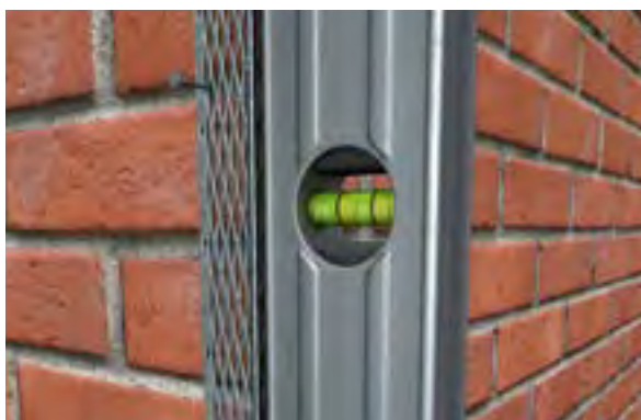
■ ENSURING THE BEAD IS PLUMB AND STRAIGHT
