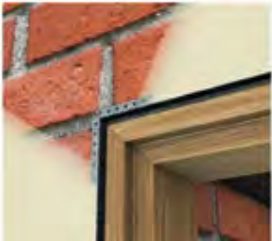
DOOR JAMB WITH SHADOW EFFECT USING R50
